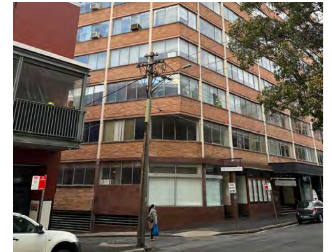
View 6. Looking east along Kippax Street
