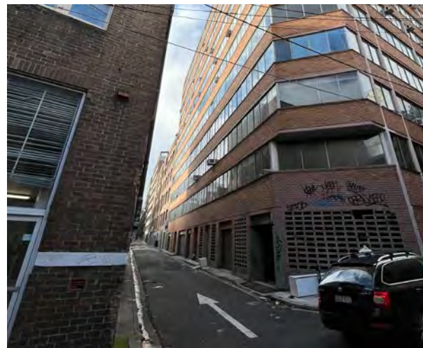
View 10. Looking south east at corner of Terry and Sophia Street
