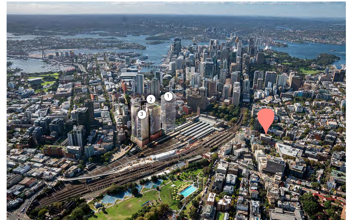
* Aerial view looking north west
