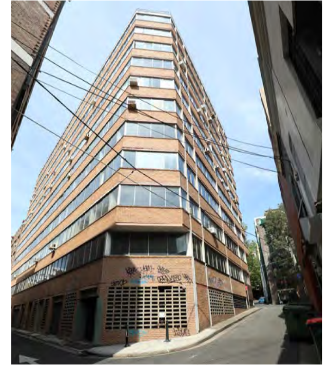
View 9. Looking south along Terry Street
