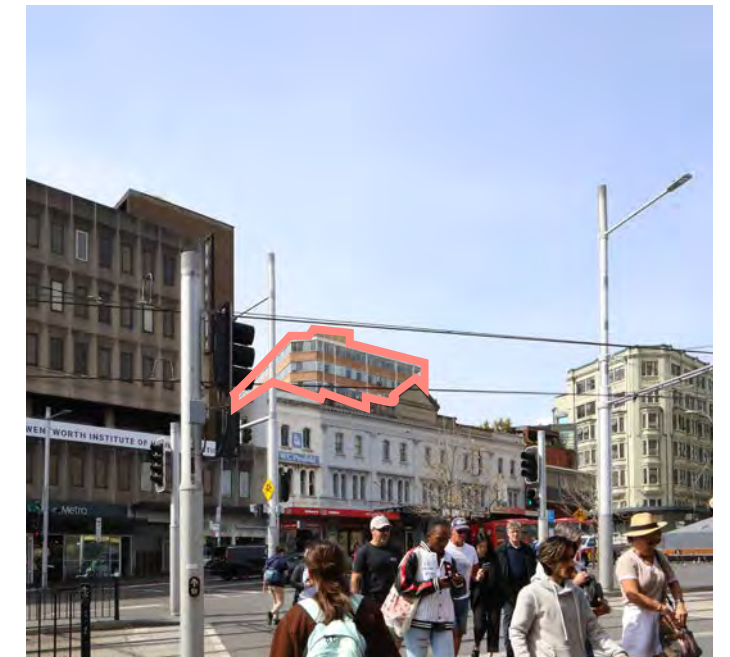
6. View towards site from intersection of Eddy Avenue and Elizabeth & Foveaux Streets looking south east
