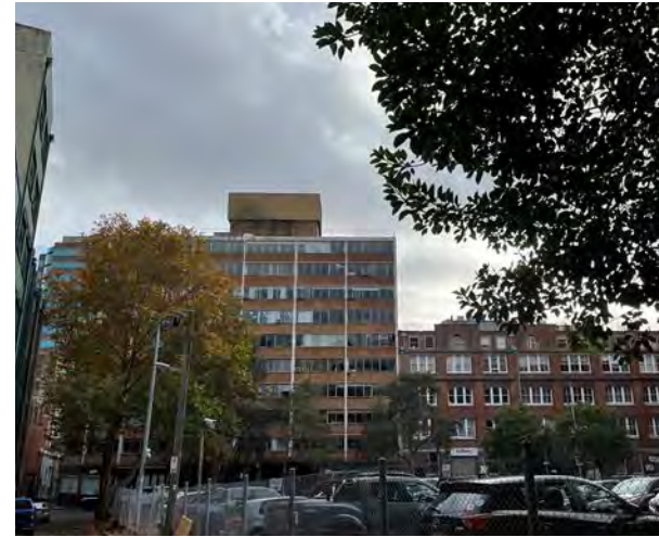
View 1. Looking North from existing carpark 19-31 Kippax Street
